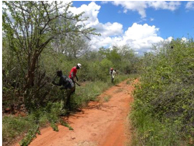
Casuals working on the Yatta road
